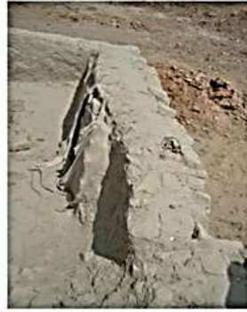
The successful use of the geo membrane, whose life is almost 100 years, this process is successfully used on the stops area, where it has been, membrane and then mud plaster is applied.
